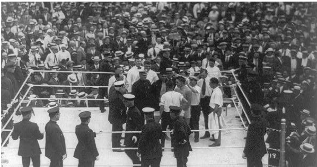
Figure 1: Dempsey and Carpentier getting ready to square off
